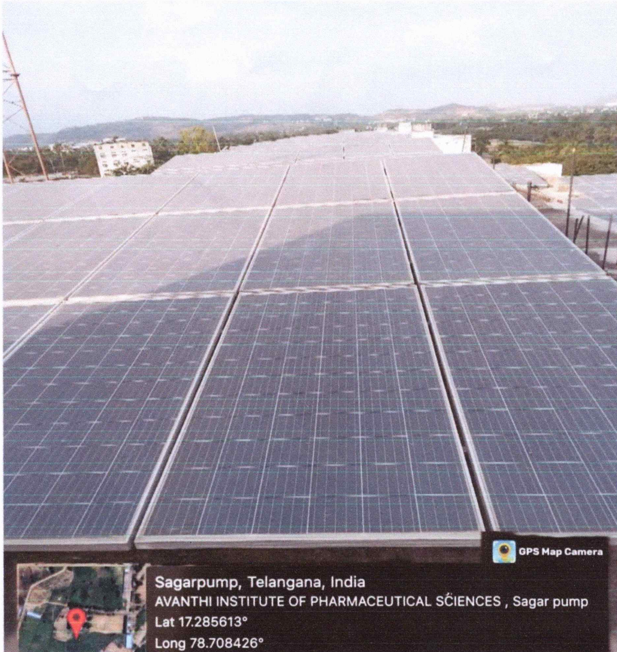
Installed solar panels on top of the Pharmacy Block-I that consist the capacity of 60 KW
